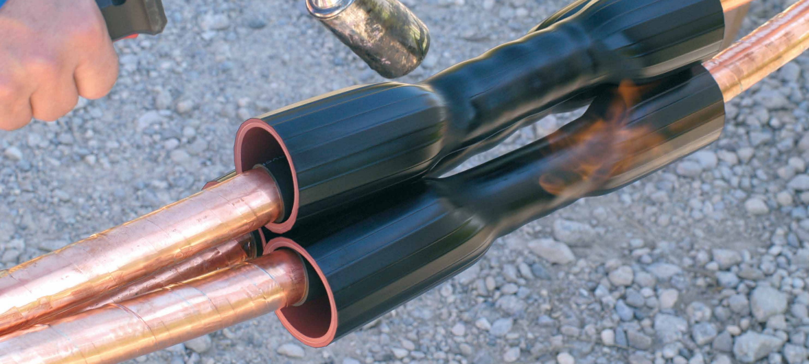
Figure Caption: Rayfit tube used in MXSU joints – Combines 3 layered, thick-wall extrusion.
